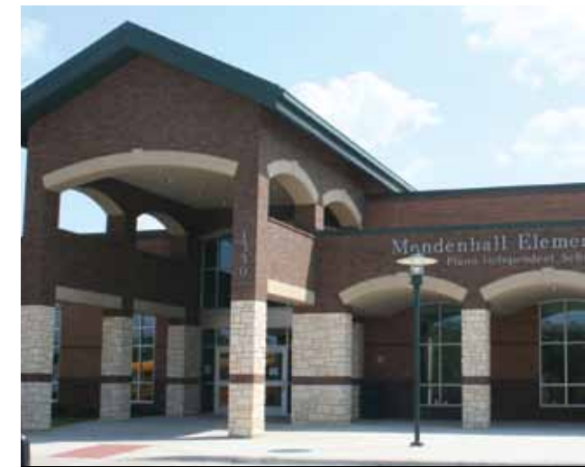
Mendenhall Elementary School was completely rebuilt with funds from the 2008 bond program on the school's original site between 18th and 19th Streets in Historic Downtown Plano.
